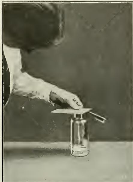
Fig. 82. Method of Introducing HNO<sub>3</sub> on Paper In Bottle In Which Sulfur Was Burned. For Preparation of Sulfuric Acid.
